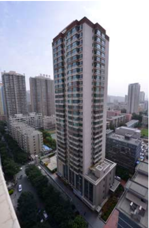
建投三号楼 NO.3 GCIGC BUILDING
